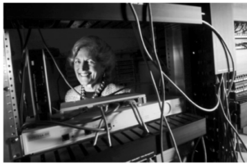
Susan Spoeher Elliott, chairman and chief executive for SSE Inc. in the newly redesigned computer server room at their office in Maryland Heights. Beck Deffenbach/Post-Dispatch
